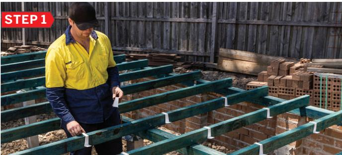
Bradford Optimo™ is most easily installed from above before the floor is installed. Place Optimo™ saddles across joists no greater than 500mm apart so to support batt from both sides, staggering the position of the saddles from joist to joist. Fasten into place using a staple, nail or screw.
