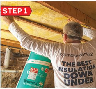
Friction fit Optimo batts tightly between the joists, as per instructions overleaf in *Installing Optimo using straps - Step 2*.
