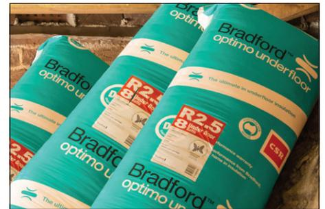
Take enough packs into the underfloor area for the whole job where possible. Start fitting insulation from the furthest point from the underfloor access.
