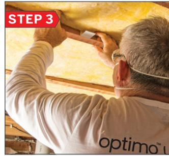
Position Optimo StayFast™ bracket on the side of joist, aligning the bottom of the bracket with the bottom of the batt. When in place apply pressure to adhere.
