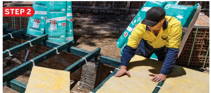
Fit insulation tightly between joists so they are resting on the feet of the Optimo™ saddle, ensuring side edges are tucked down adjacent to the joist so not to impede adhesive used to fix flooring on joist. Do not leave any gaps between insulation. Flooring can be installed once the insulation is in place.
