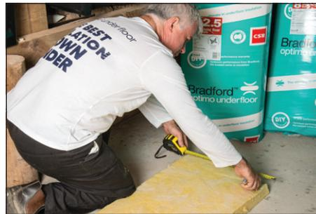
Switch off power at the fuse box. Measure your floor joist spaces. Usually 450mm centres or 600mm centres. For 450mm centres use 415mm wide batts. For 600mm centres use 565mm wide batts. Trim batts with knife if too wide.
