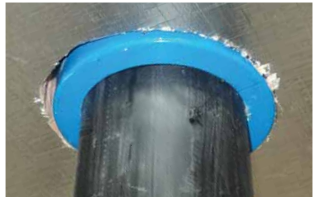
Figure 7 Penetration example - Kingspan Kooltherm® K10 PLUS Soffit Board installed tight around the fire collar and HDPE service pipe.
